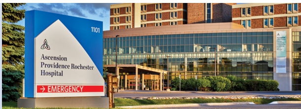
Ascension Providence Rochester Hospital
